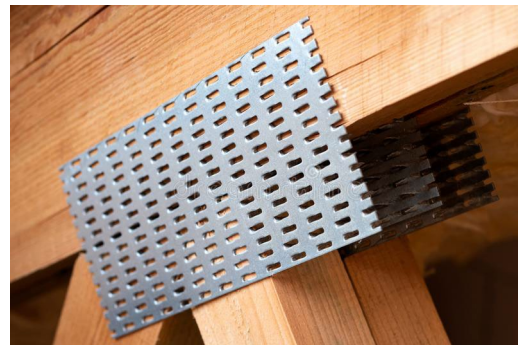
Figure 3. Detailed truss with galvanized nail plate.
