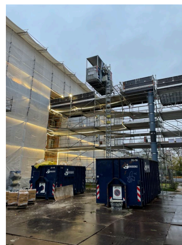
Figure 2: Façade scaffolding and platform between Buildings
